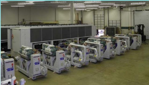
Chilled Water systems are normally closed loop networks. Make up water is minimal and resulting mainly from leaks. Therefore the main problem that is found in these systems is corrosion and metal dissolution. If the system is left untreated metallic surfaces would be subjected to pitting and general corrosion due to dissolved ions and electric potential.
