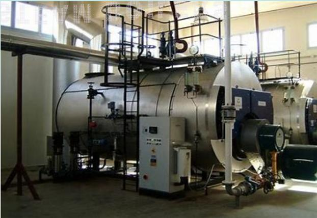
It's very important and essential for the boiler to be well-protected against scale depositions on steel tubes' surfaces in order to maintain good heat exchange efficiency and prevent the losses in fuel & energy.
