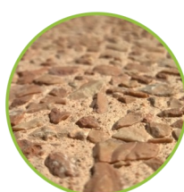
Medium exposure. Exposure depth approx. 2.5 mm
